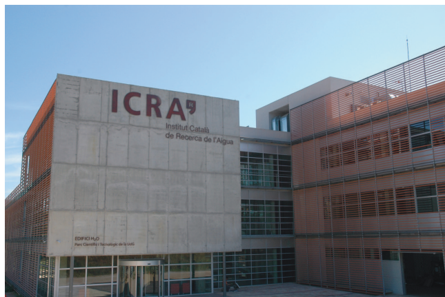
Fig. 1. External view of the ICRA's H2O building.
